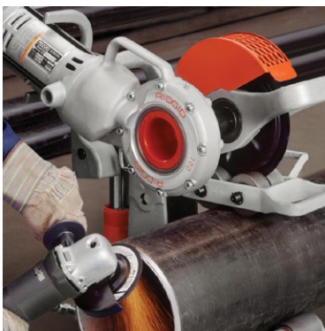
Model 258 with Pipe Roller in use for beveling. Two operators are recommended for this operation
